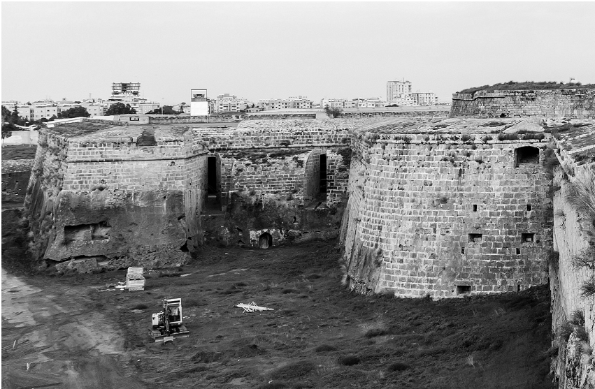
Figure 2.3 Famagusta: The south flank of the Martinengo bastion. The San Luca bastion is centre right. Visible are the internal square gunports on two levels and the arched port of the flanking embrasure in the parapet. In the centre can be seen the southern postern gate of the Martingno bastion between the deep embrasures of the piazza bassa.
