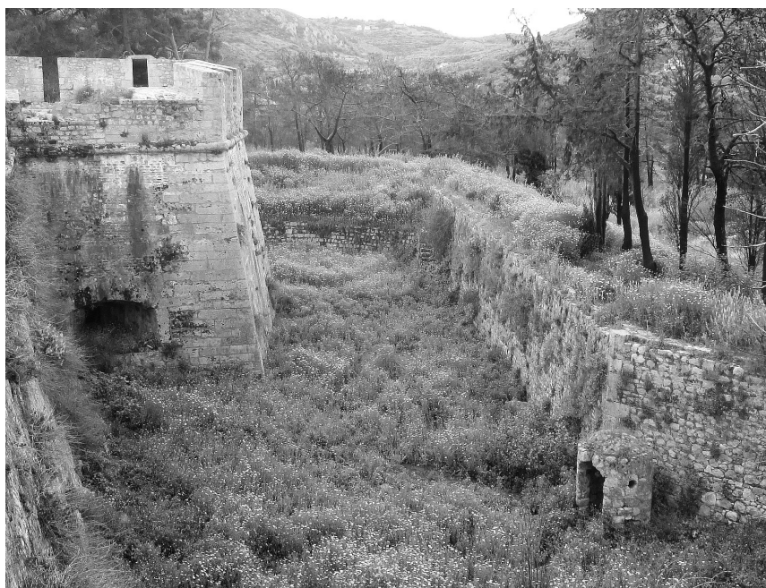
Figure 6.27 New Navarino: The southwestern section of the ditch showing the counterscarp and steeply sloping glacis. In the flank of the Citadel's southern bastion is the arched opening of a Turkish gunport. A domed sentry box is visible lower right.
