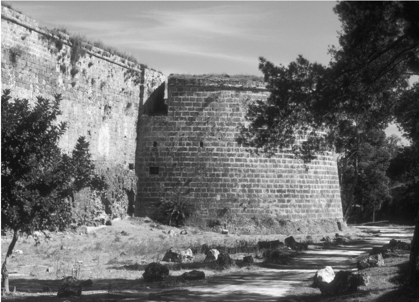
Figure 2.1 Famagusta: The west flank of the Santa Napa bastion. The deep flanking embrasure in the parapet and the square gun port of the internal chamber are visible.
