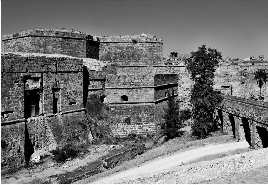
Figure 2.2 Famagusta: The Land gate complex. Visible are the gate in the southeast flank of the ravelin, the Turkish screen wall connecting the ravelin to the curtain, and the Turkish bridge. Behind these structures can be seen the bulk of the high cavalier.
